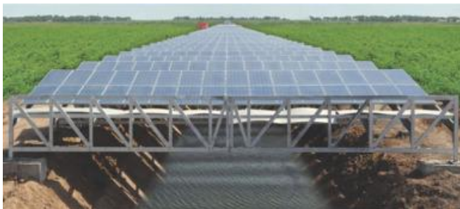
Canal top solar systems.
