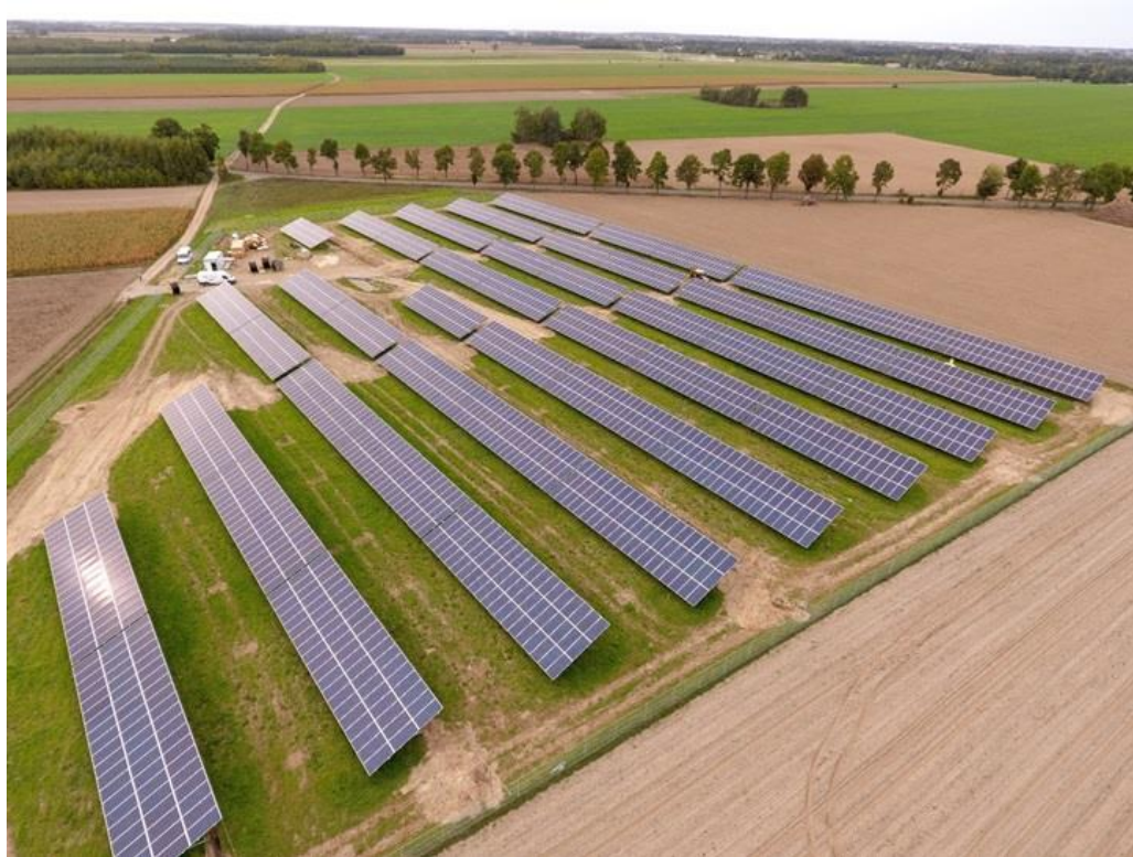
Power plant 1MW in Pluskocin
